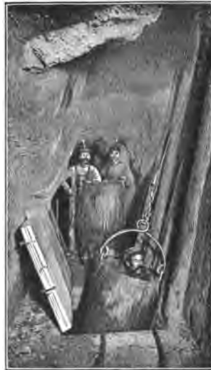
Elevator in Mine.
